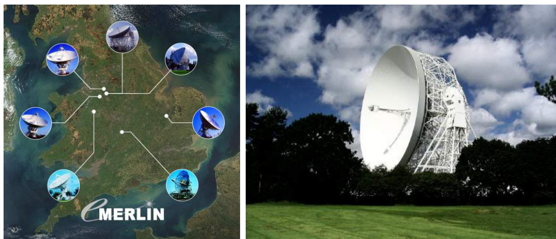
Figure 5.2: e-MERLIN interferometer - Left: The seven dishes from e-MERLIN are, clockwise from north, Jodrell Bank Lovell, Jodrell Bank Mark II, Cambridge, Defford, Knockin, Darnhall and Pickmere. Right: The Lovell Telescope, with 76.2 m in diameter, is the third largest fully steerable radio telescope in the world. Credit: Jodrell Bank Centre for Astrophysics, University of Manchester (e-MERLIN image) & Anthony Holloway, Jodrell Bank Centre for Astrophysics (Lovell picture).
